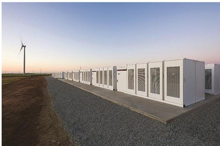
*Tesla 100 MW Powerpack battery storage system integrated into the 99-turbine, 309 MW Hornsdale Wind Farm located in Jamestown, South Australia and developed by John Laing and Neoen.*
